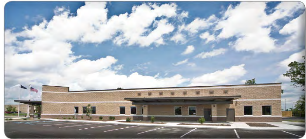
Monitoring Operations Center—Anderson Indiana 24 Hours a Day/7 Days a Week/365 Days a Year
