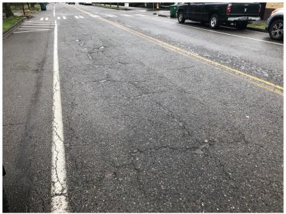
Skyway Area: Deteriorating pavement, upheaved, narrow sidewalks – old infrastructure beyond designed lifespan.
