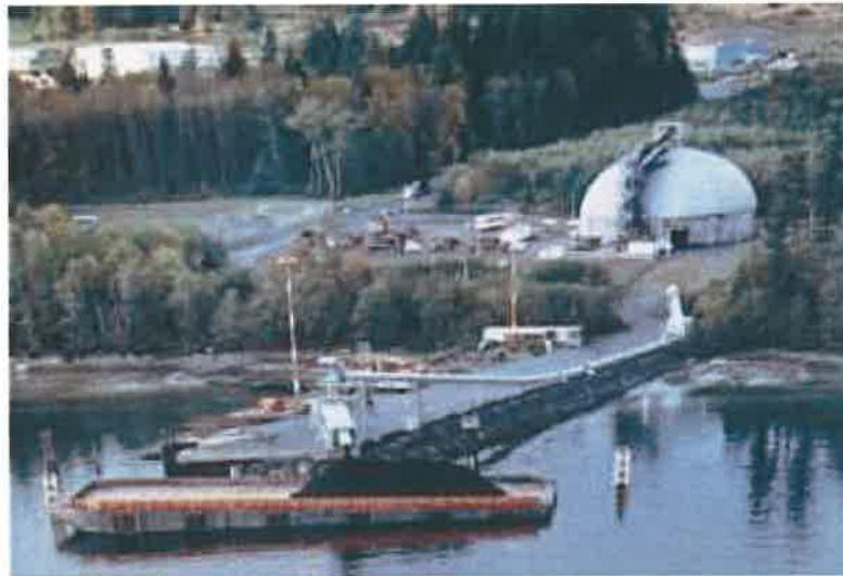
Figure 7: Middle Point Barge Loading Facility (Dome Storage in Background)
