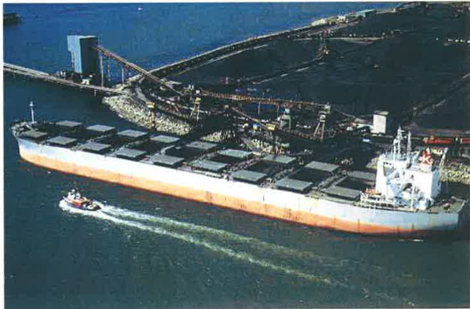
Figure 2: Berth 2 with Dual Quadrant Shiploaders
