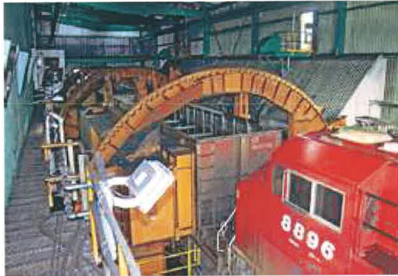
Figure 3: Rotary Railcar Dumper
