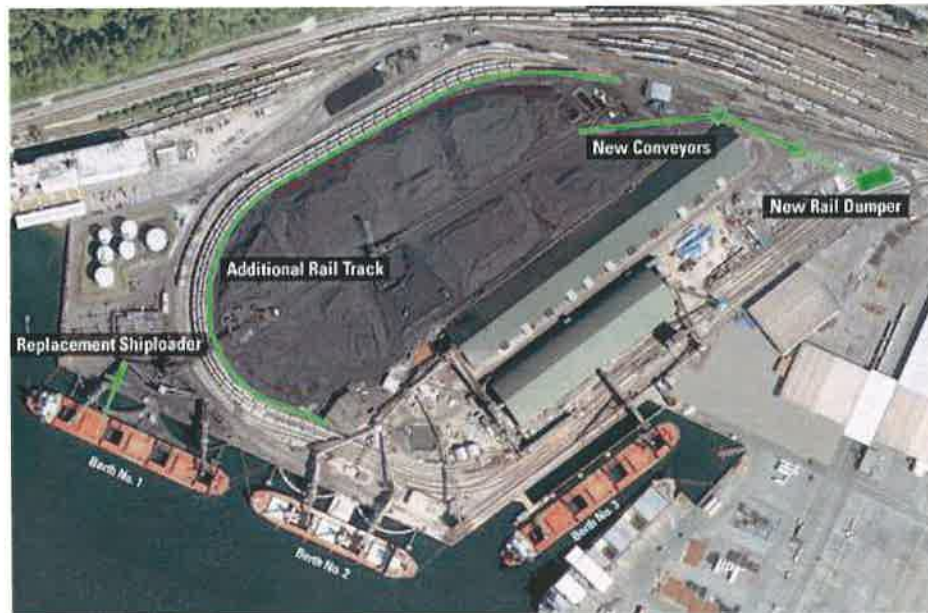
Figure 6: View of Improvements to the Coal Handling System.
