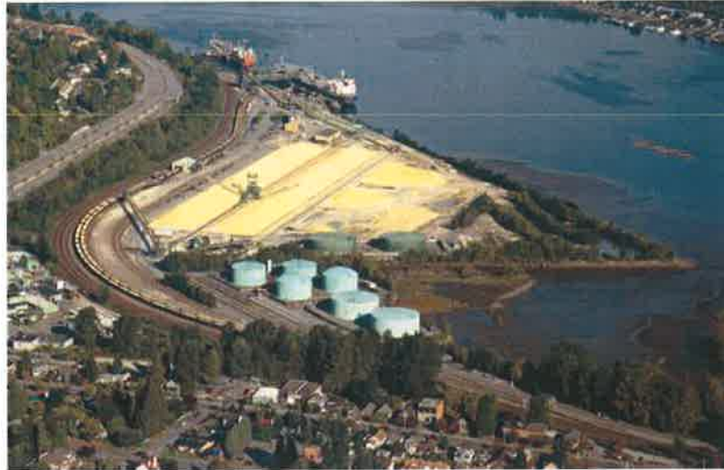
Figure 14: Aerial View of Pacific Coast Terminals
