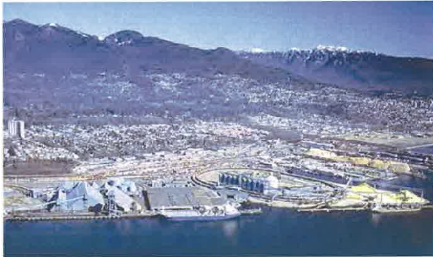
Figure 12: View of Vancouver Wharves – Looking North
