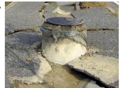
Manhole floats from liquefaction
