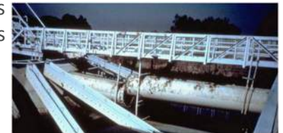
Damaged clarifier
