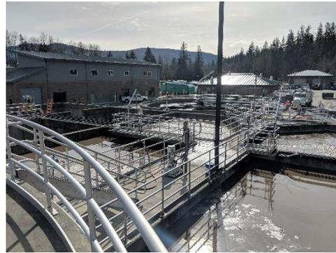
*WRF Oxidation Ditches and Solids Handling Building*
