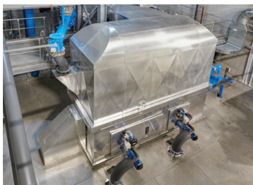
▲ Dryer hood with sludge feed
