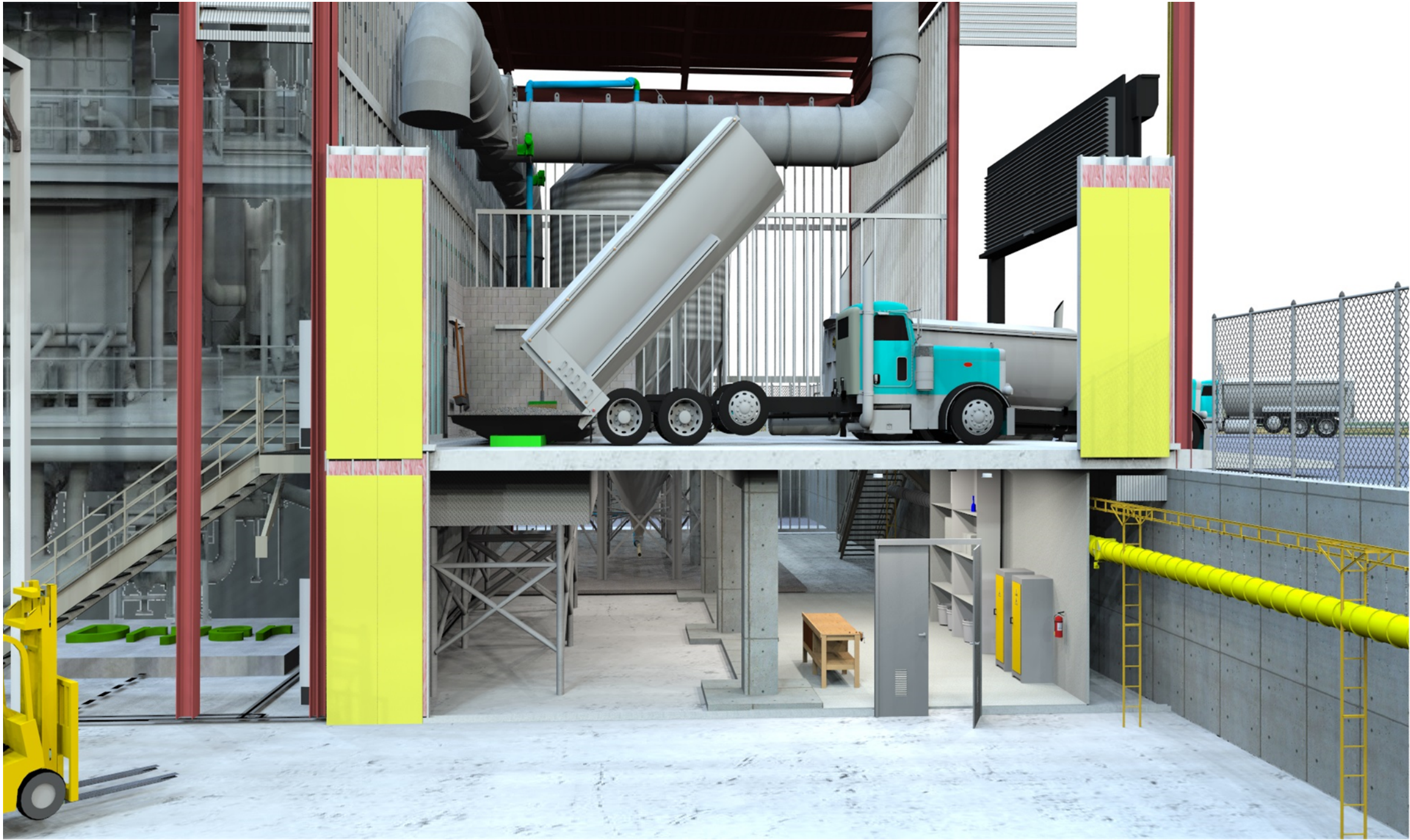
Dryer Building - Wet Sludge Receiving
