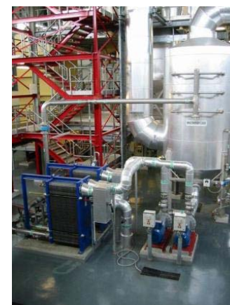
Spray Condenser with heat recovery pumps and heat exchangers (up to 75% heat recovery as hot water)
