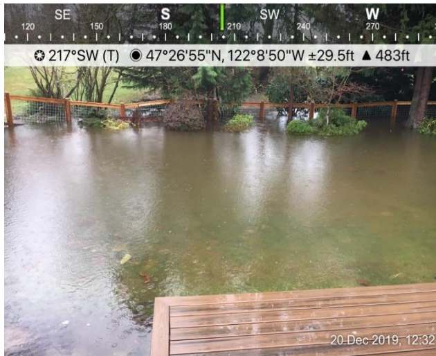
Photo 2: Looking southwest at the backyard of 14609 SE 173rd St.
