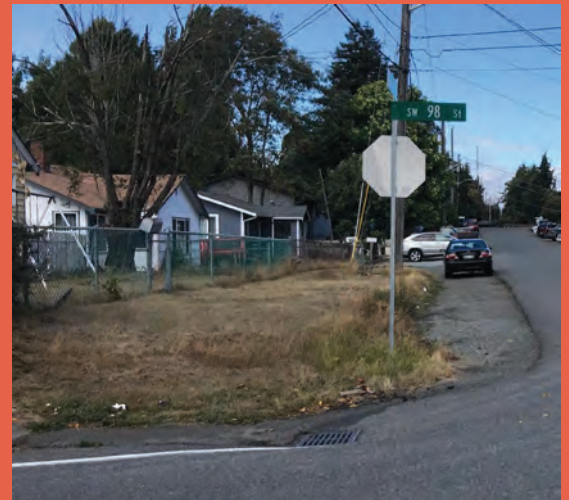
Drainage runs to catch basins via gravel street edges
