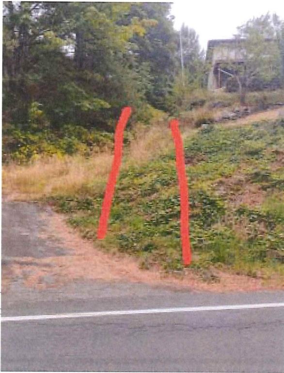
1. Looking up the undeveloped unmaintained roadway from S Star Lake Rd. that is causing erosion of 2 parcels- #796760-0140 and #735100-0180 *at 27 Degree Slope*
