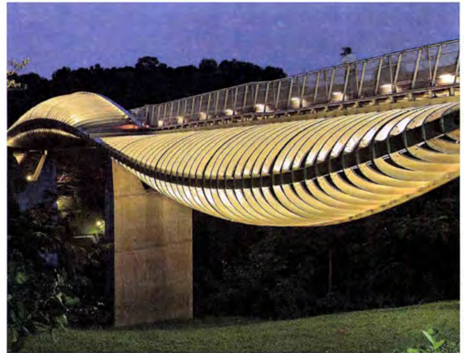
Henderson Wave Bridge – Singapore
