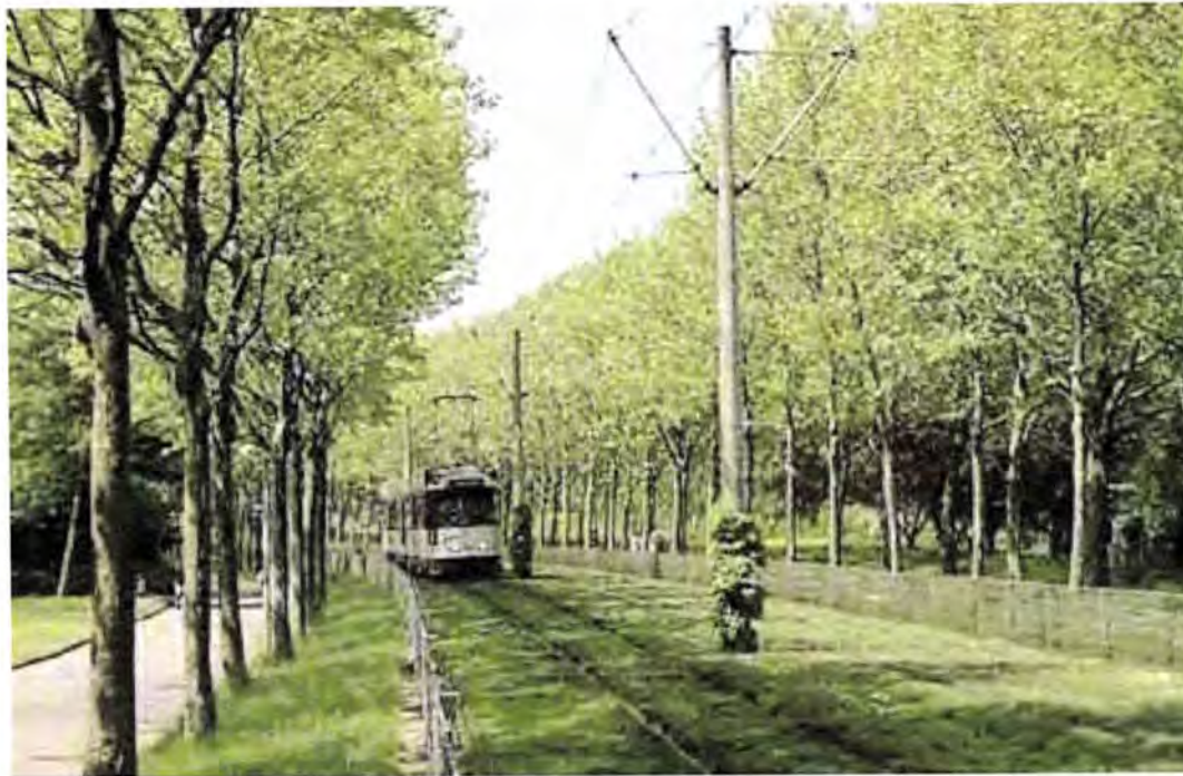
VAG Tram System and Trail – Freiburg, Germany
