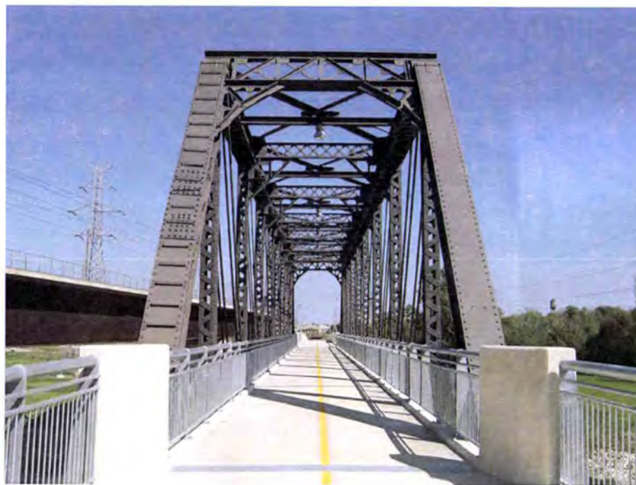
Santa Fe Trestle – Santa Fe, NM
