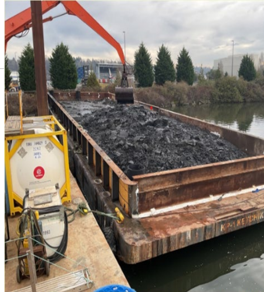
A barge holds excavated sediment from Sediment Management Area (SMA) 6.
