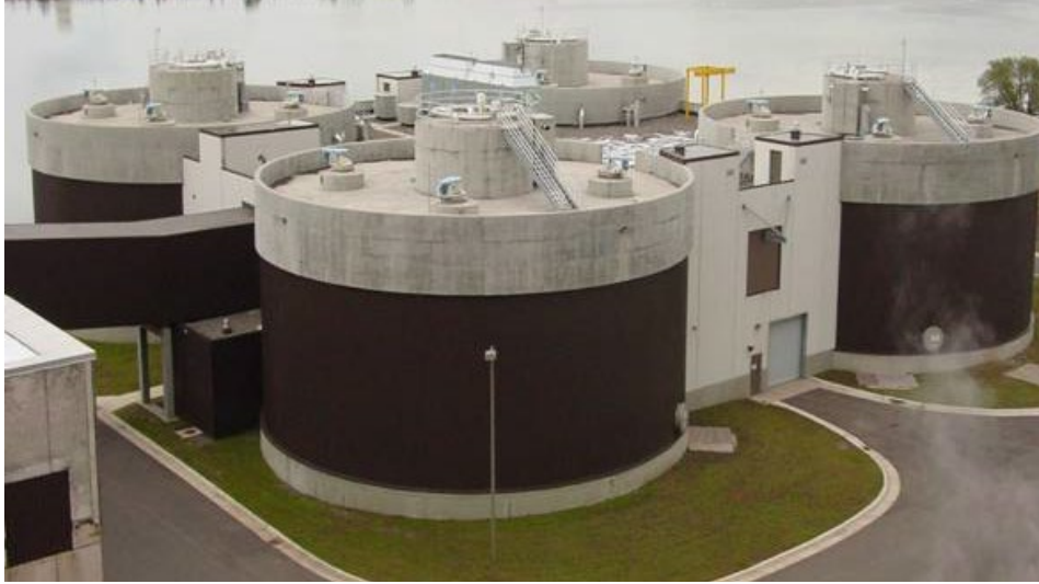
Figure 2. TPAD at Western Lake Superior Sanitary District WWTP
