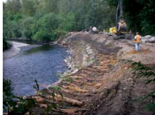
Levee project funded by the King County Flood Control District
