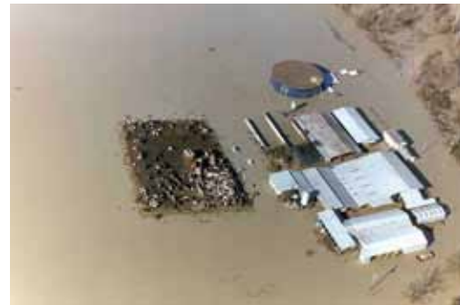
Farm pads. Roughly two dozen farm pads have been constructed in flood-prone agricultural areas of King County since the early '90s, and another dozen are under construction as of 2012.
