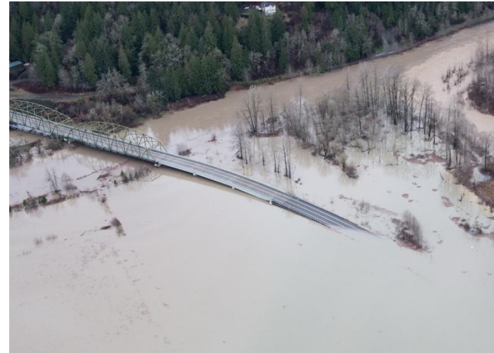
Tolt Hill Road inundated
