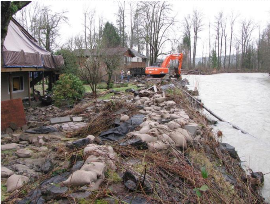
Tolt River emergency repair Jan. 2009
