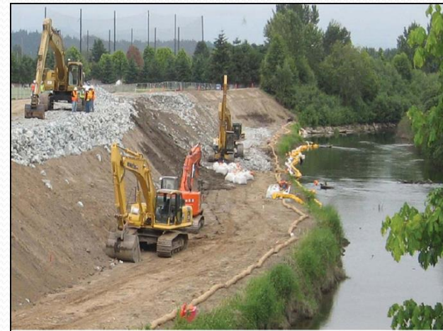
Example of levee reconstruction adjacent to river (Green River)
