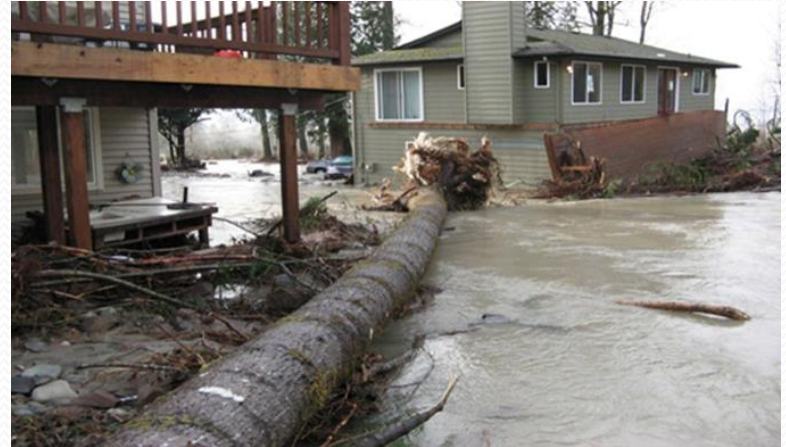
Levee breach (Tolt 1.1)
