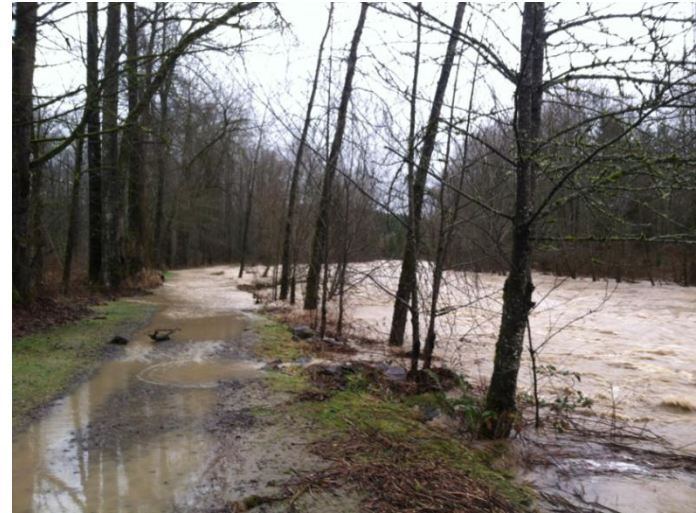
Frew levee overtopping
