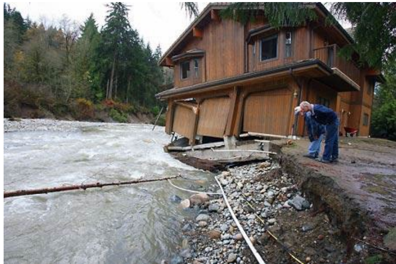
House destroyed due to channel migration along the Raquin River.
