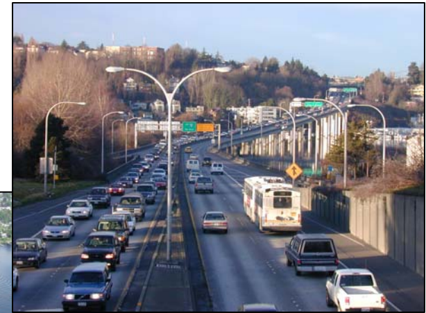
Portage Bay Bridge – Facing West
