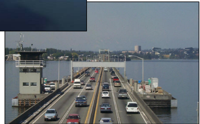
Midspan of the Floating Bridge – Facing West
