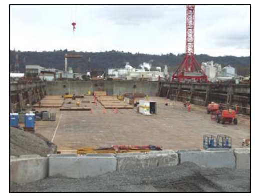
Hood Canal Bridge pontoon construction site, Concrete Technology, 2006
