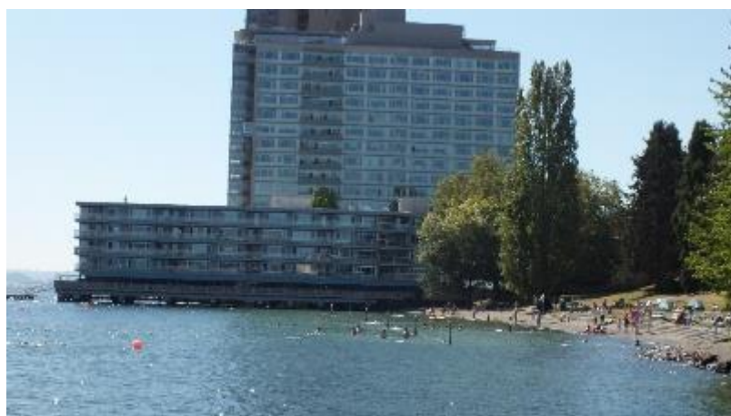
Figure 10- Madison Park as seen from the existing dock, looking south
