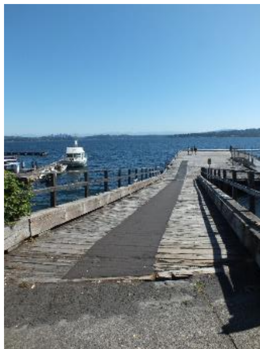
Figure 14- View of the Leschi Park site, looking east
