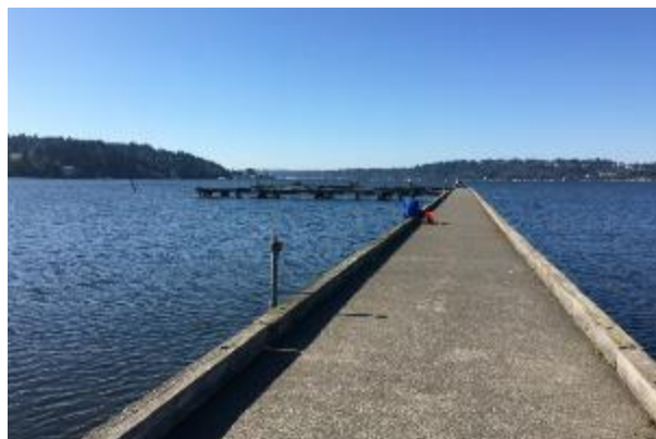
Figure 6- View of the Log Boom Pier, looking southwest
