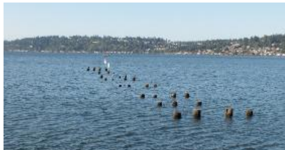
Figure 5- Pile field south of Log Boom Pier
