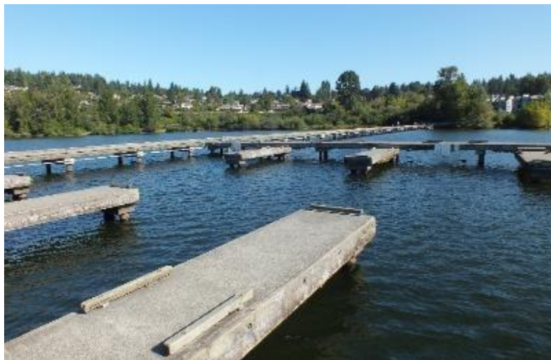
Figure 4- View of the finger piers and Log Boom Park, looking north
