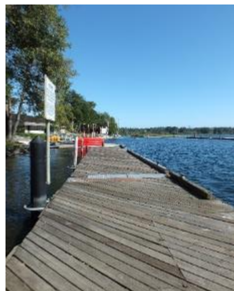
Figure 8- Dock at UW landing site, looking north
