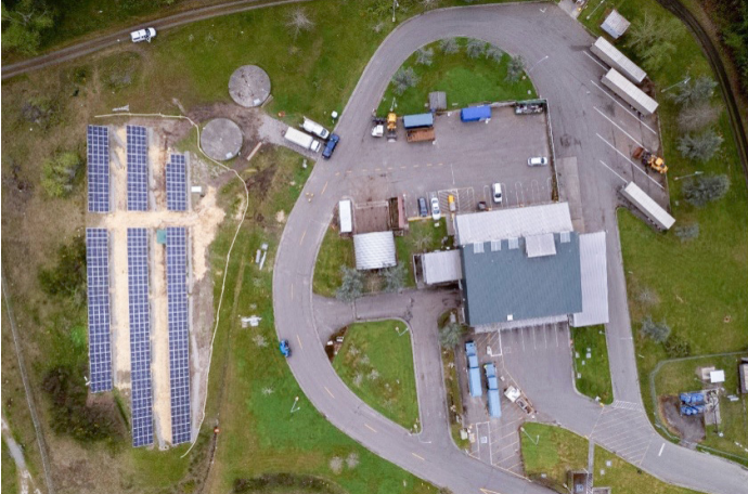
The Solid Waste Division worked with local installer Western Solar to build the new array – a connected network of 348 solar panels – on previously unused land next to the Vashon transfer station.
