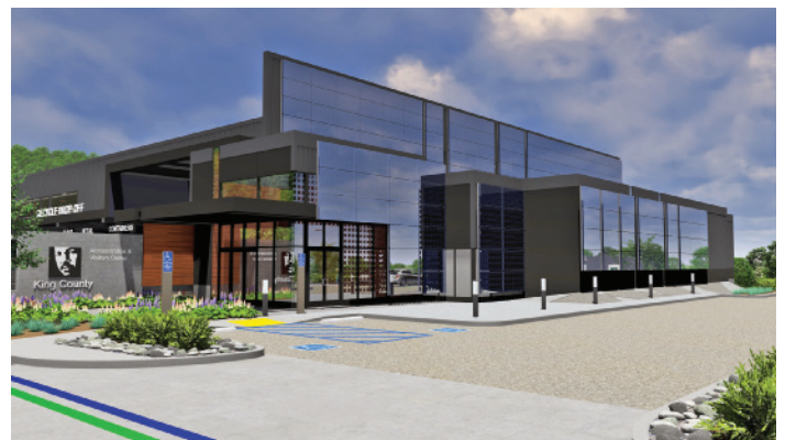
The Division is modernizing its services to include increased recycling options in areas of King County that are underserved. Pictured is a conceptual design of the South County Recycling and Transfer Station coming to Algona in 2026.
