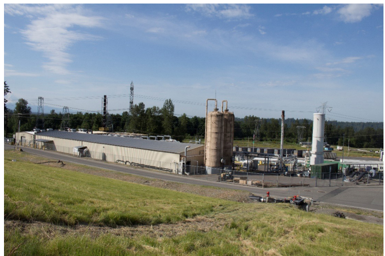
The onsite Bio Energy Washington facility processes landfill gas into a renewable energy source.
