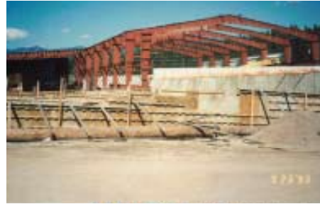
Distant view of the central portion of the main building frame
