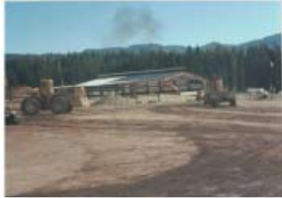
Distant view of skelton building
