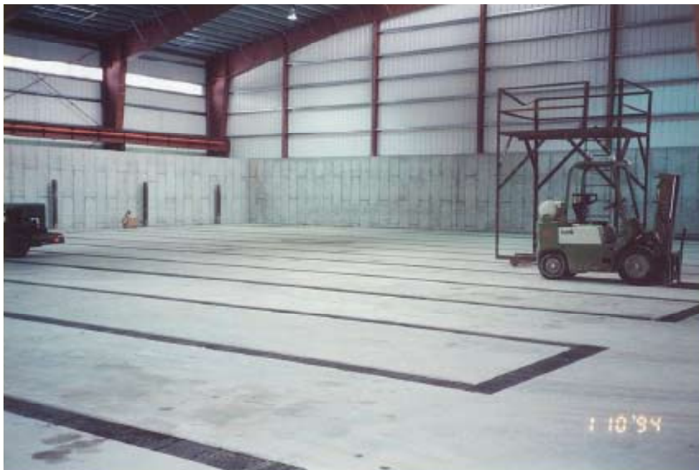
Aeration floor unit
