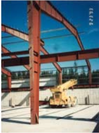
Main building under construction view
