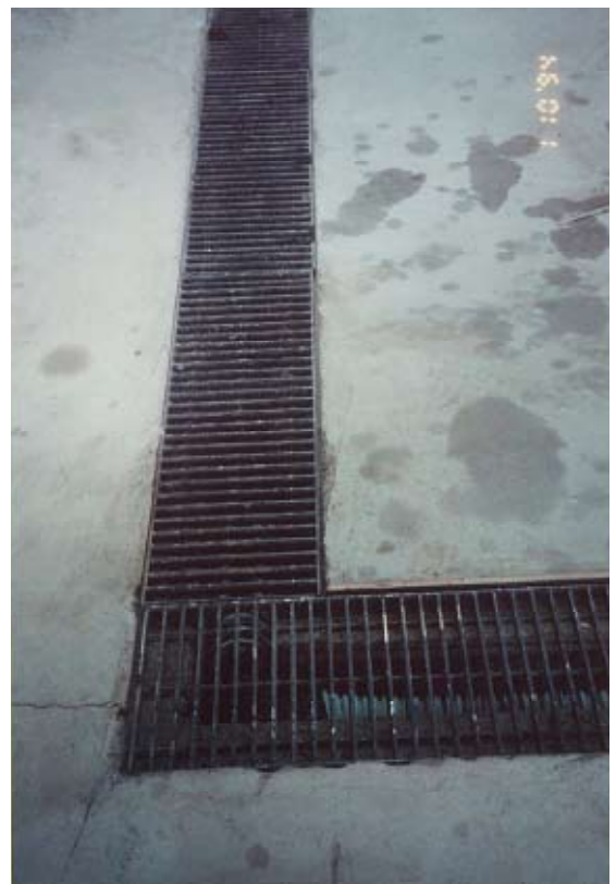
Aeration floor unit
