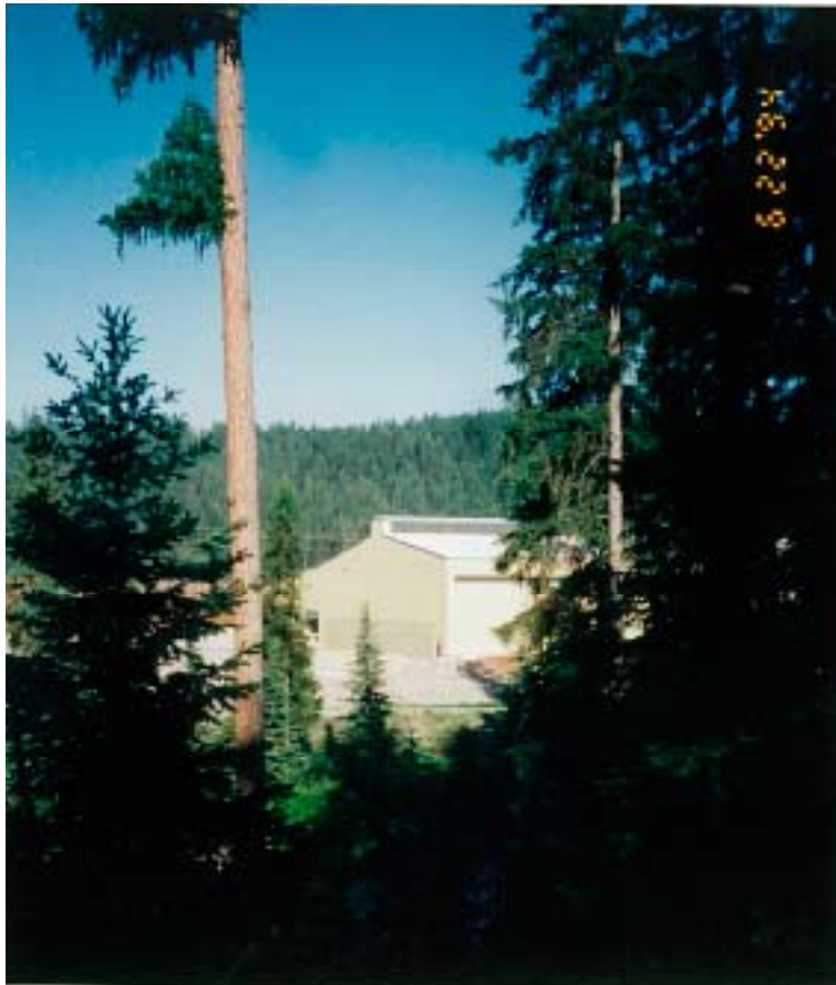
Olney Montana, nestled in a forested area. This building is 285 feet by 180 feet and 42 feet high
