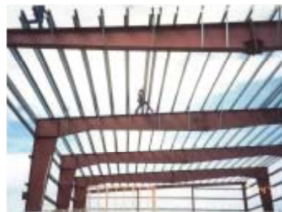
Main building roof framing
