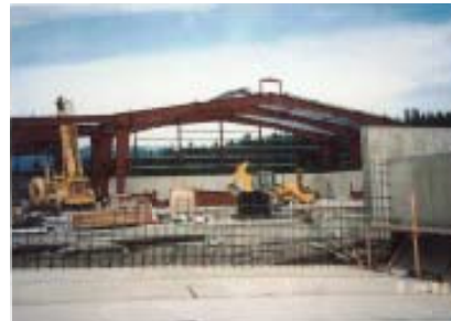
Main building under construction view
