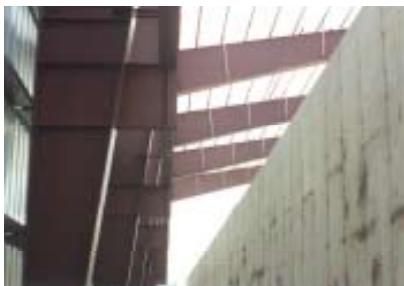
Interior walls and passage way for computer room and infrastructure piping etc
