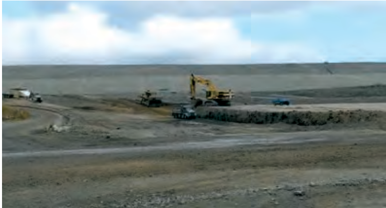
Developing a new area requires extensive excavation and preparation
