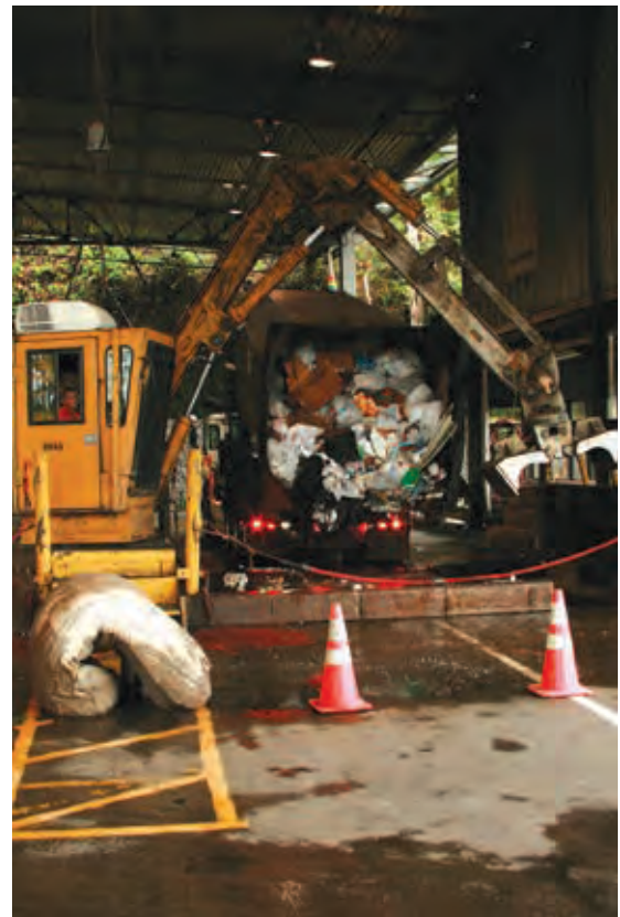
The Algona Transfer Station was built in the mid-1960’s
