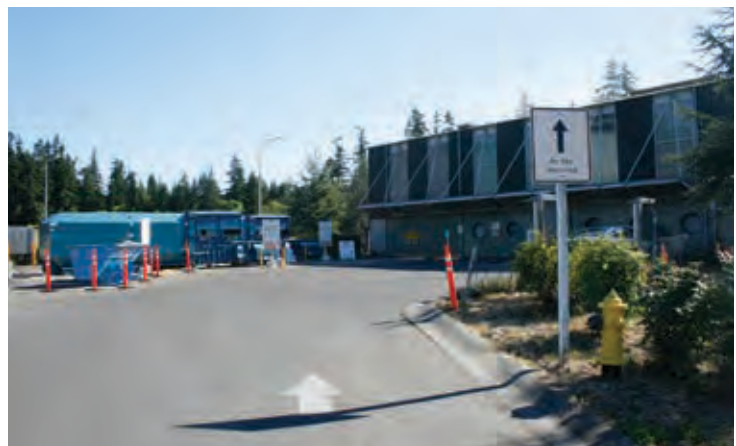
The Vashon Recycling and Transfer Station
