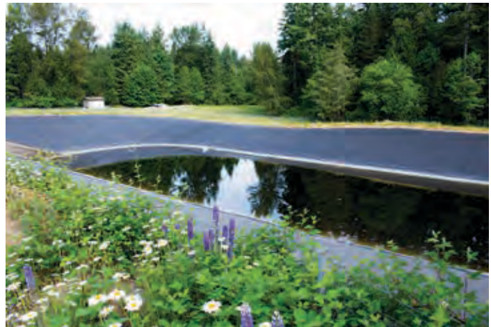
A stormwater pond at the Cedar Hills Landfill II is part of the infrastructure paid for by the Facility Improvements Account
