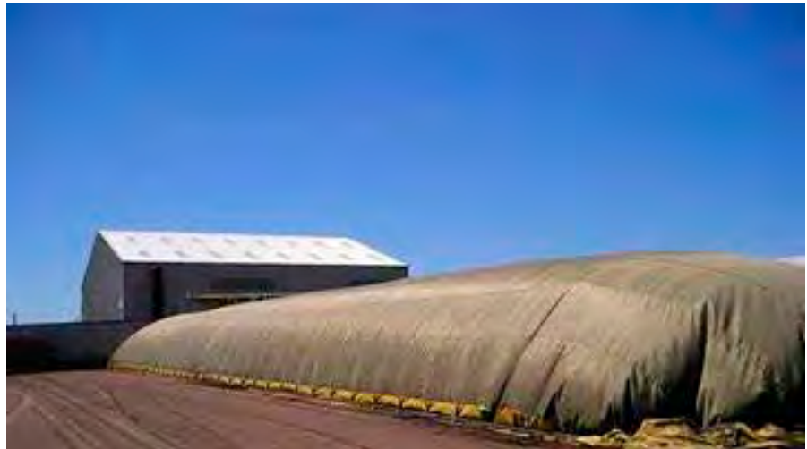
Cedar Grove Composting Facility (Photo courtesy of Cedar Grove)
