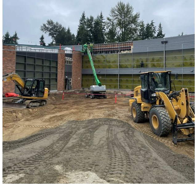
Redmond Middle School Addition
