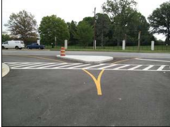
A restricted right-in, right-out example.
