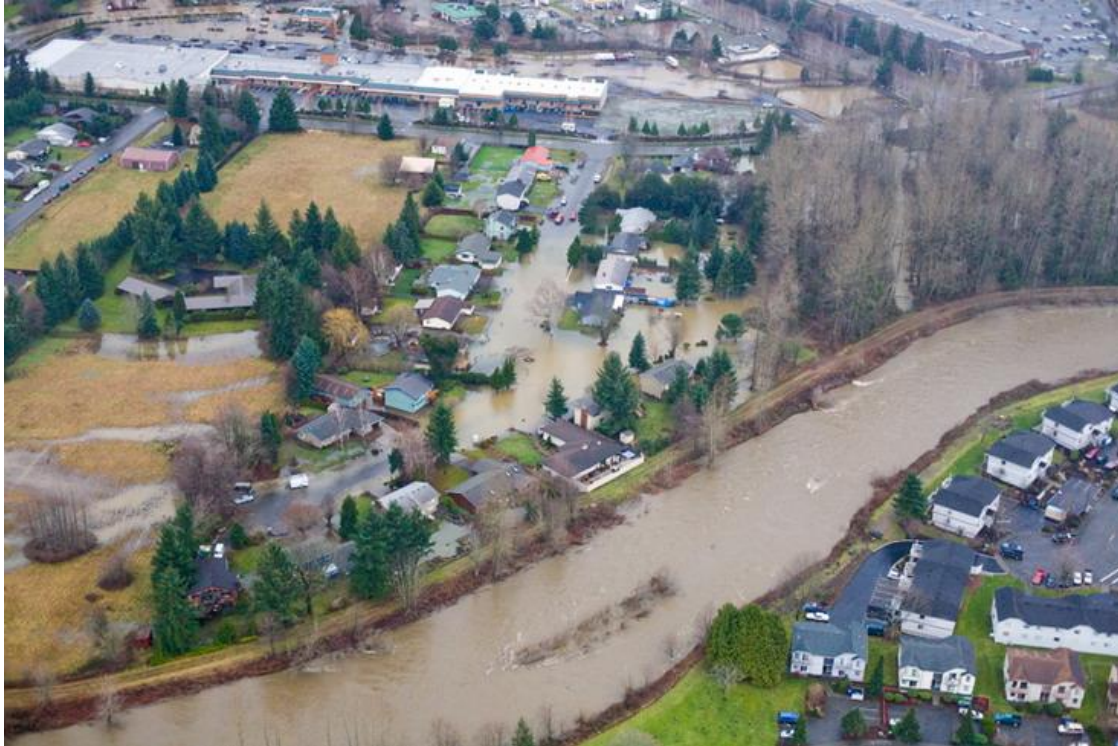
Snoqualmie River at 413th Avenue SE (Shamrock Park). January 7, 2009.
