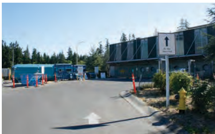
The Vashon Recycling and Transfer Station
