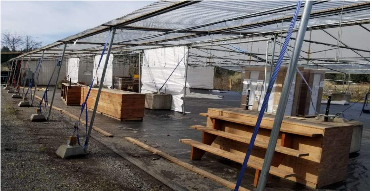
Above: Temp Tent tie downs south side
