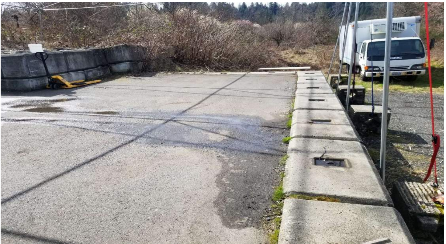
Below: Loading dock looking west
