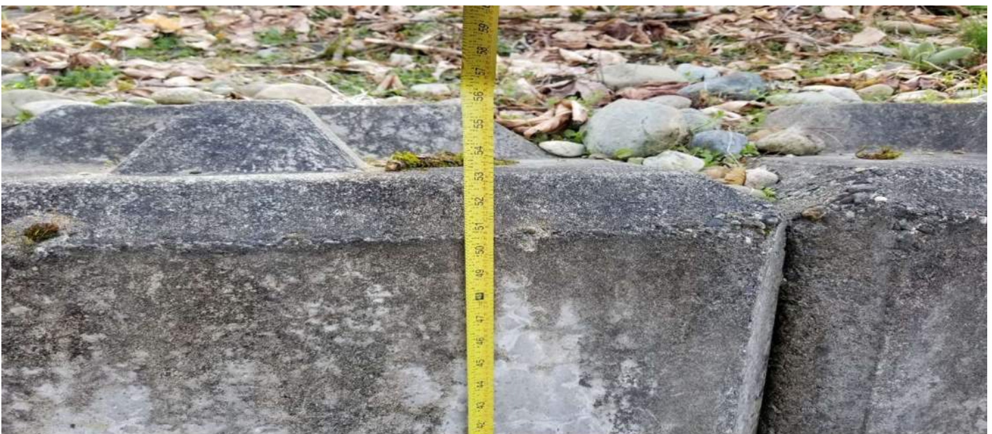
Below: Ecology Block wall (2 Blocks High) 53" tall
