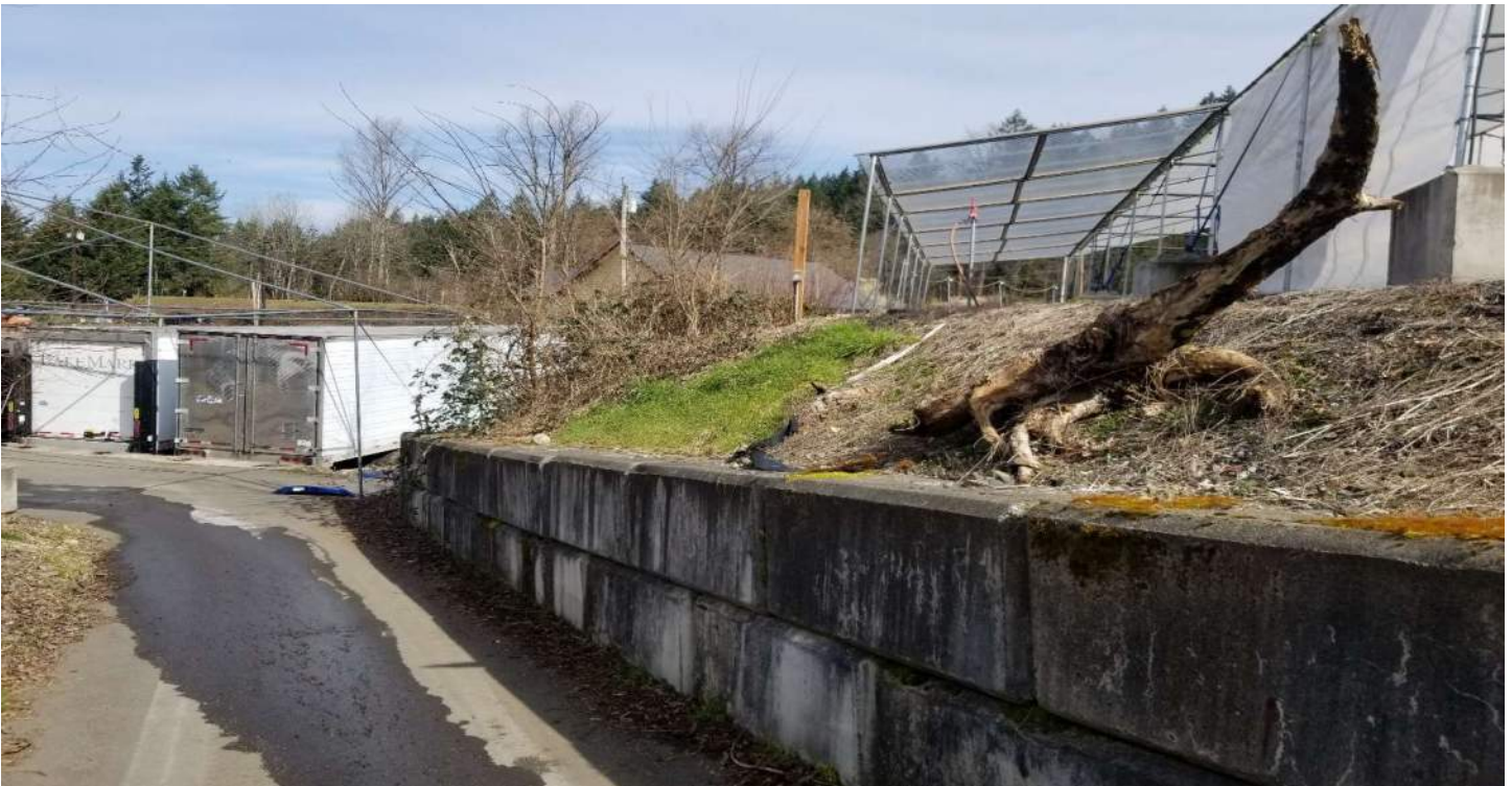
Below: 10' wide asphalt path to loading dock and eco block wall looking north
