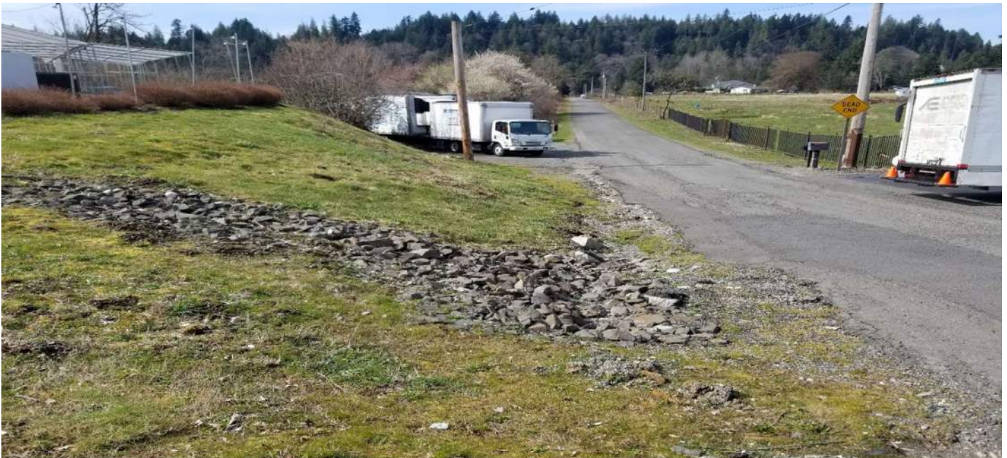
Below: Looking at Rip rap pad where lot drains to as well as CB in eastern parking lot
