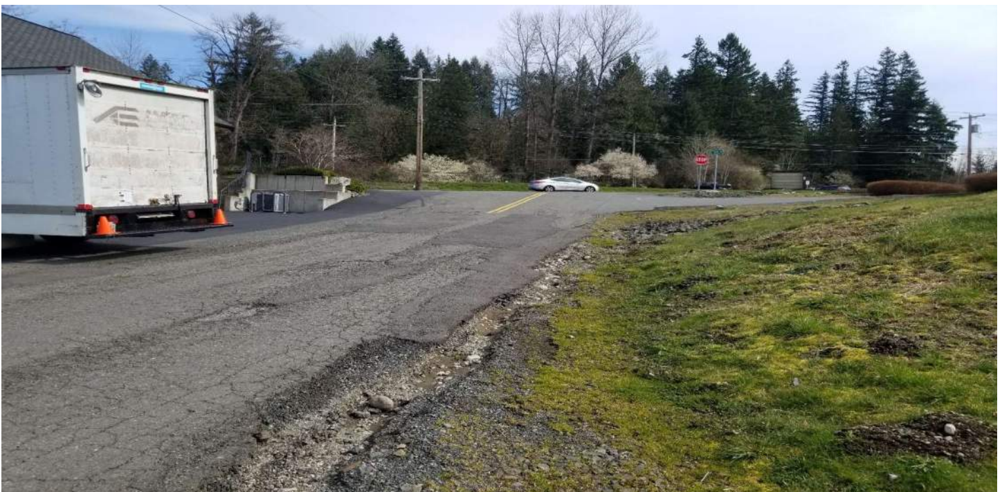
Below: Looking north at driveway access and storm drain out fall
