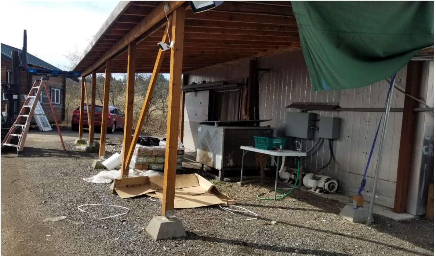
Above: Freezer unit south side of building
