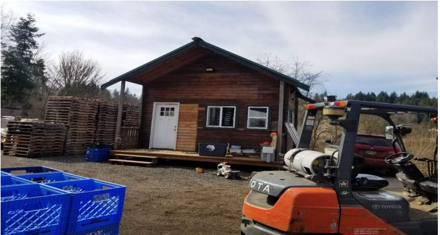
Above: Office Building east side of structure
