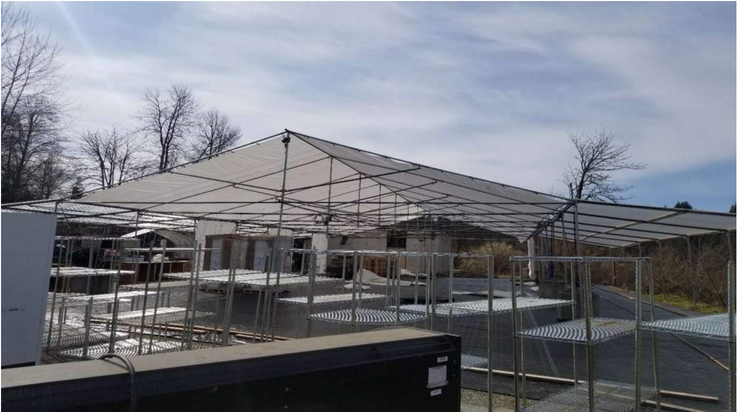
Above: Looking at Temp Tent structure
