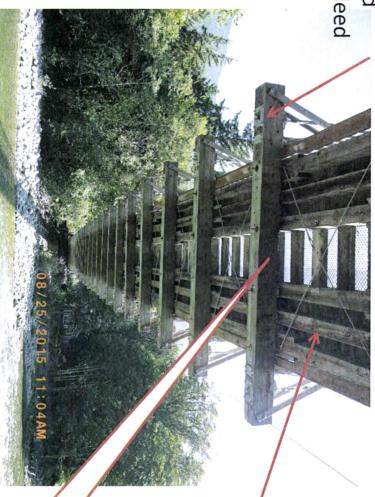
All stringers were sounded and drilled at two different locations on the main span. More than 40% of these stringers were found very soft at top and bottom. Some have splits or crushing
