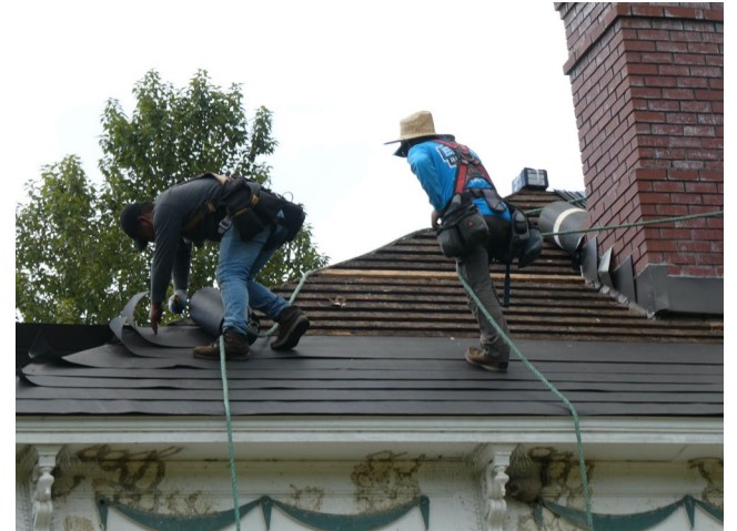
Neely Mansion restoration in action, new overlapped felt-paper rolled out on top of original skip jack boards. Photo: Linda Van Nest
