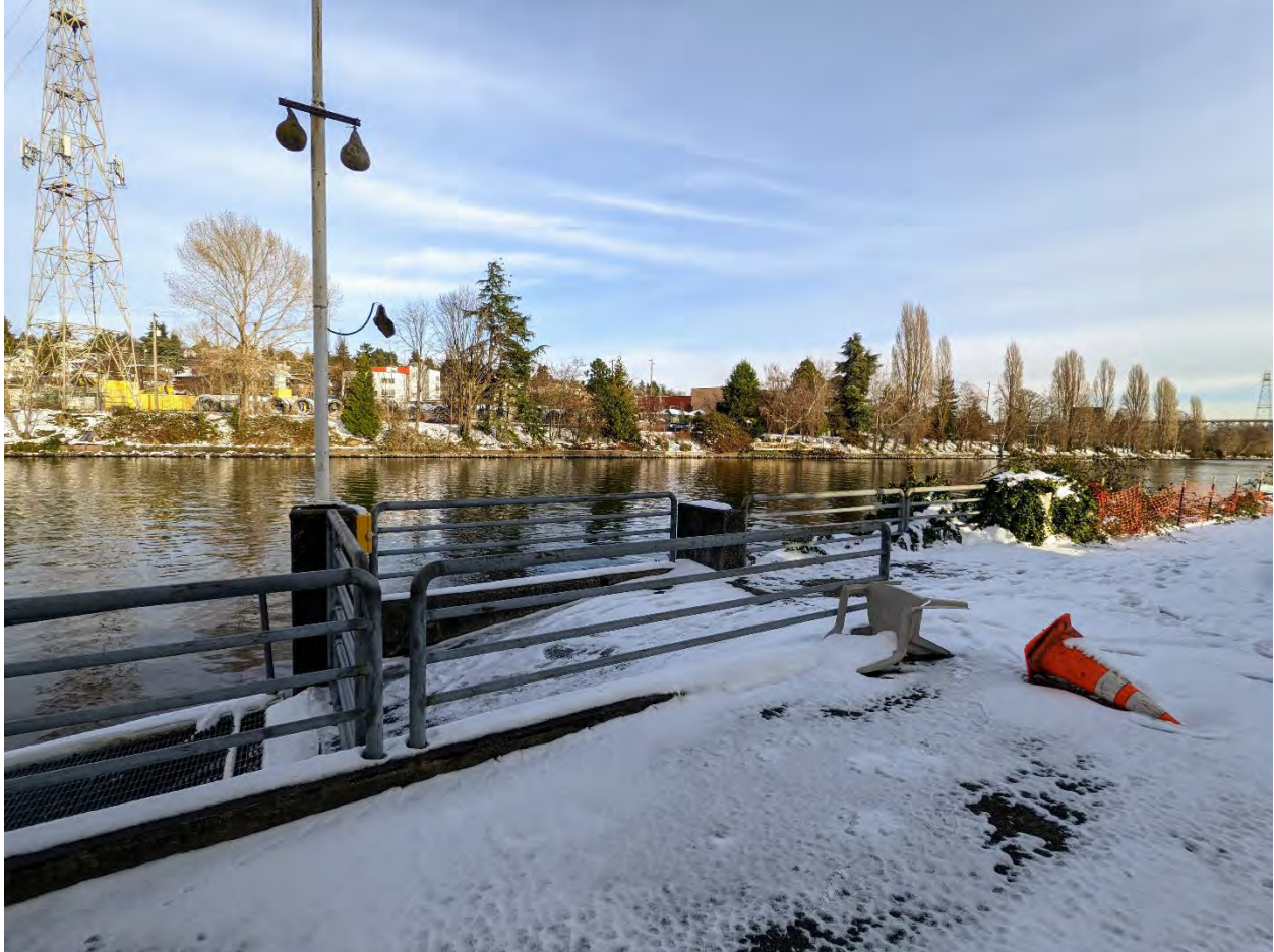
Figure 5 – King County bulkhead lease area (looking SE – taken 29-DEC-2021)
