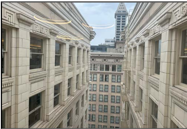
Outlooks through one of three light wells, photo facing south. Courtyard Hotel in the background, with views of Smith Tower.
