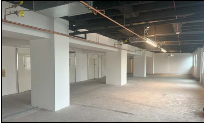
View of upper floor shell vacant space.
