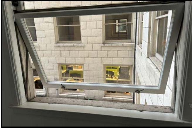
View of operable windows and outlooks facing light well.
