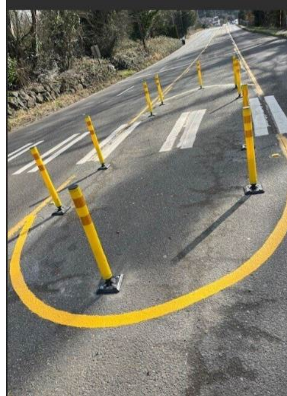
Roads installed 13 traffic calming “islands” on Renton Ave to calm traffic and prevent unsafe passing
