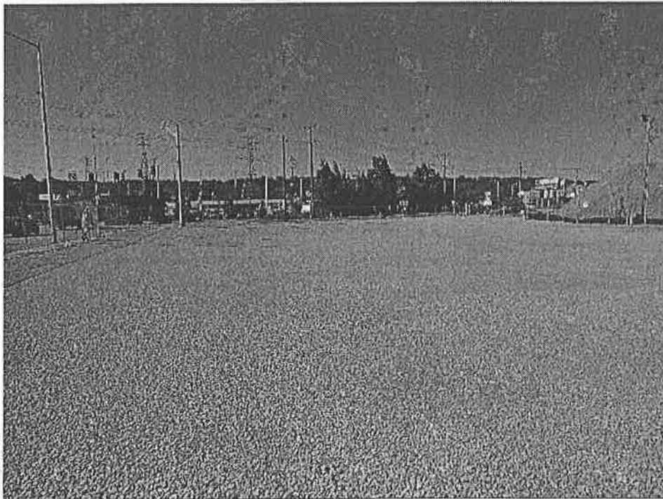
Preconstruction view of project site looking west
