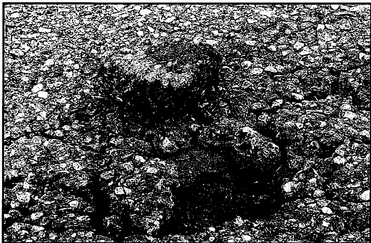
Figure 6: Representative of pavement degradation generating FOD.
