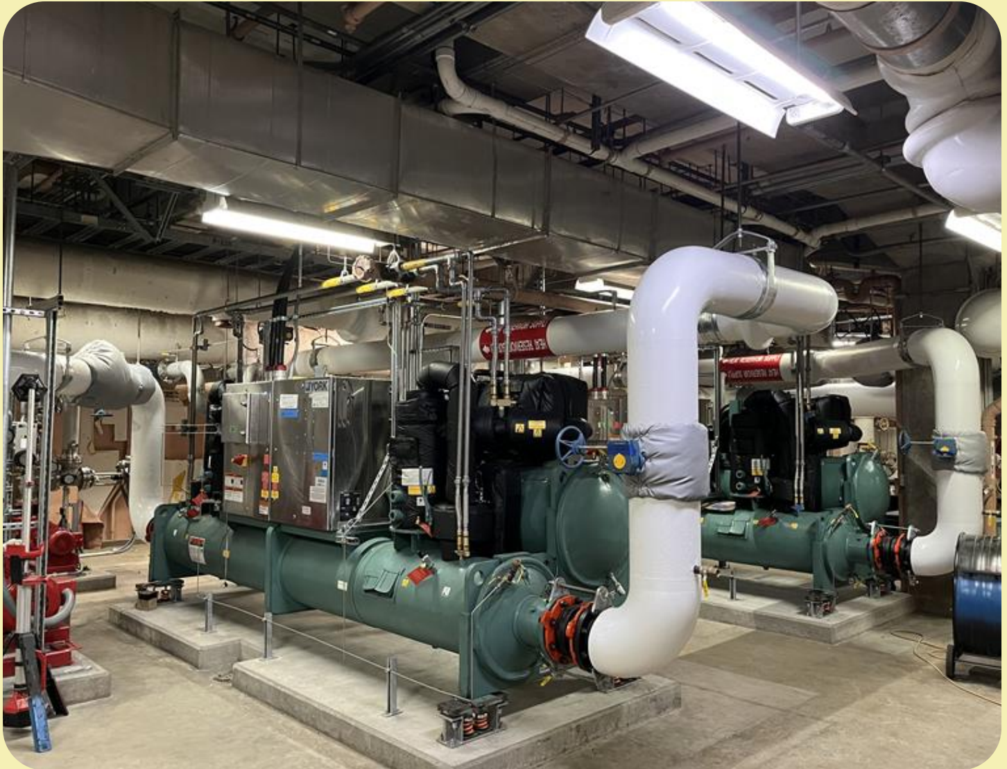
New industrial heat pumps at the South Wastewater Treatment Plant are significantly reducing natural gas usage.
