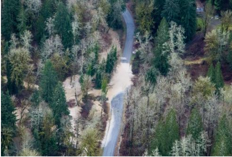
Tolt River Road inundated
