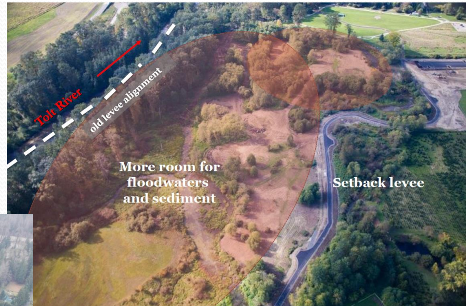
Lower Tolt River Floodplain Reconnection Project
