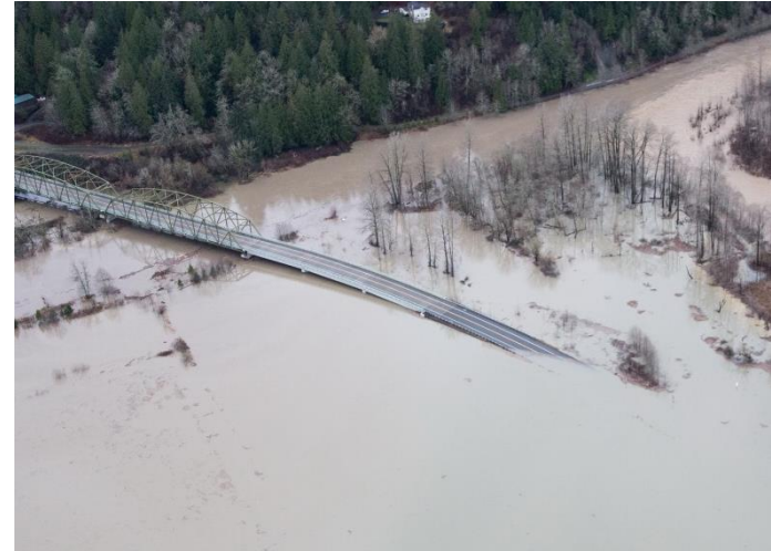
Tolt Hill Road inundated
