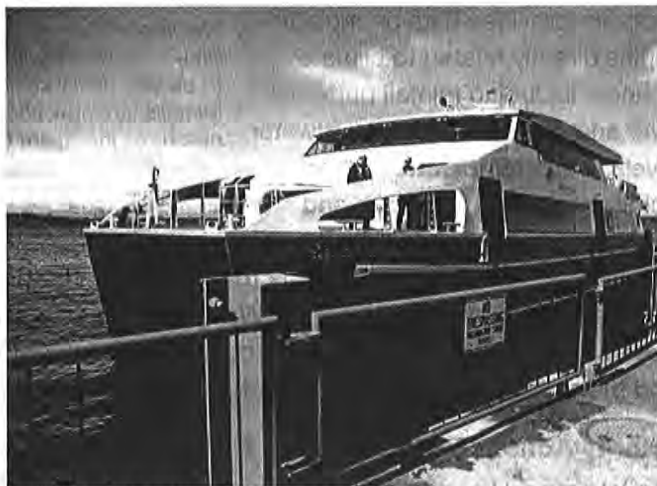
Floating docks used by the Water Taxi are attached to pilings, with floating gangways attached to neighboring fixed docks.
