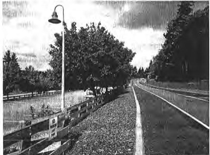
A stretch of NE Novelty Hill Road project near Perrigo Park that includes porous asphalt shoulders and Low Impact Development strategies.
