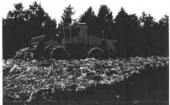
Compacting garbage at the Cedar Hills Regional Landfill
