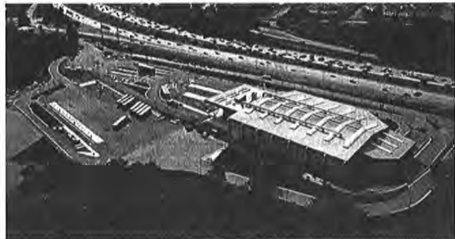
Solid Waste Division's Bow Lake Recycling and Transfer Station located in Tukwila achieved a LEED Platinum level certification featuring renewable energy, water reclamation and reuse system, and Forest Stewardship Council (FSC) certified wood.
