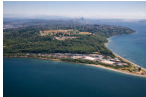
West Point Wastewater Treatment Facility on the edge of the Puget Sound. King County is incorporating the latest science about rising sea levels into planning and operations of the wastewater treatment and conveyance system.
