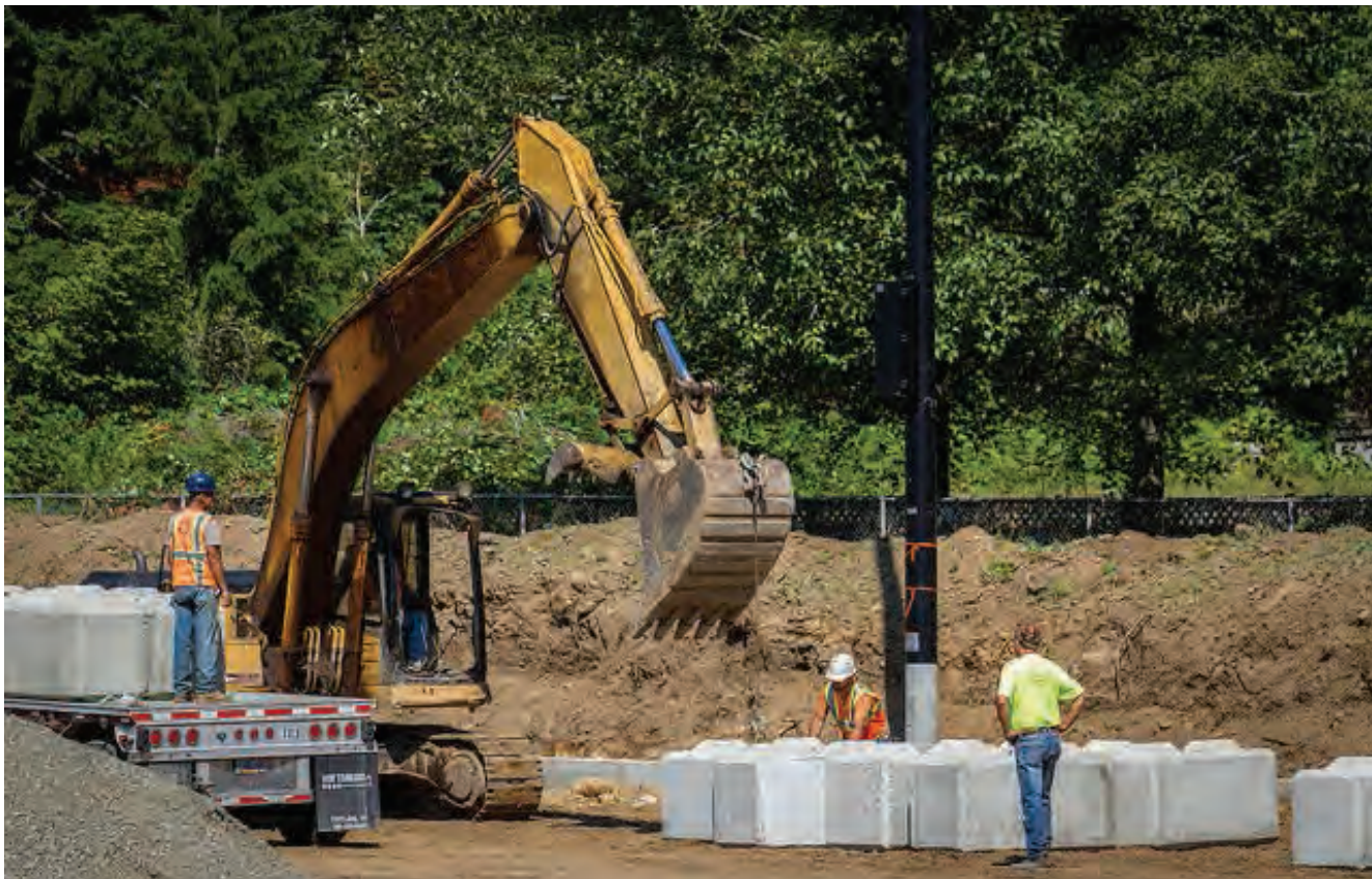
Preston Ballfields Construction
