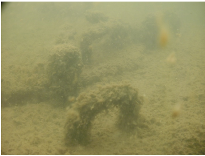
Photograph 7. Manhole 35 lifting eye.
