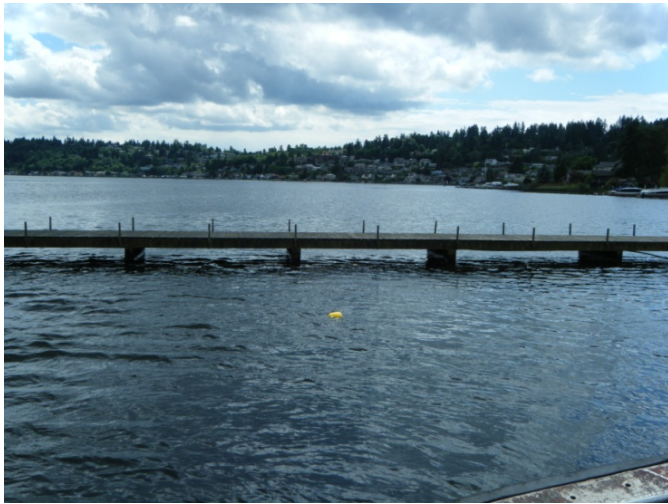
Photograph 9. Facing south at Manhole 35.
