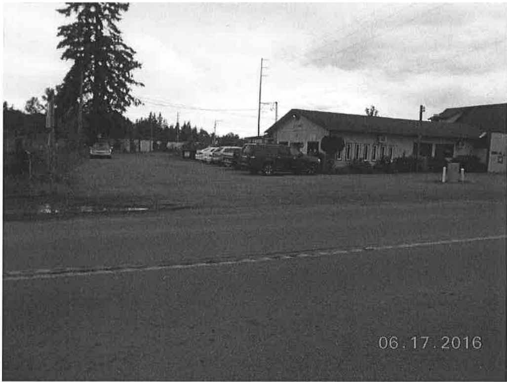
Photo 2: Looking north at the buildings and west parking area. The septic system is behind the white fence in the background.
