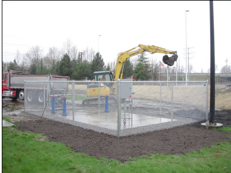
Work completed on the Sewer Lift Station at the MRJC
