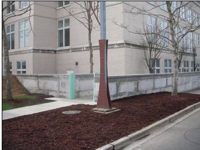
Ecology block wall on North East Corner of MRJC
