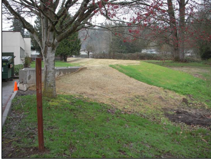
Completed berm at Aukeen District Court
