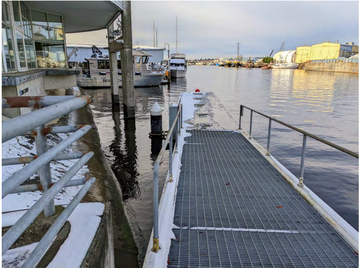
Figure 3 – King County bulkhead lease area (looking NW – taken 29-DEC-2021)
