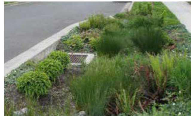
A rain garden designed to treat stormwater runoff in a residential area.
