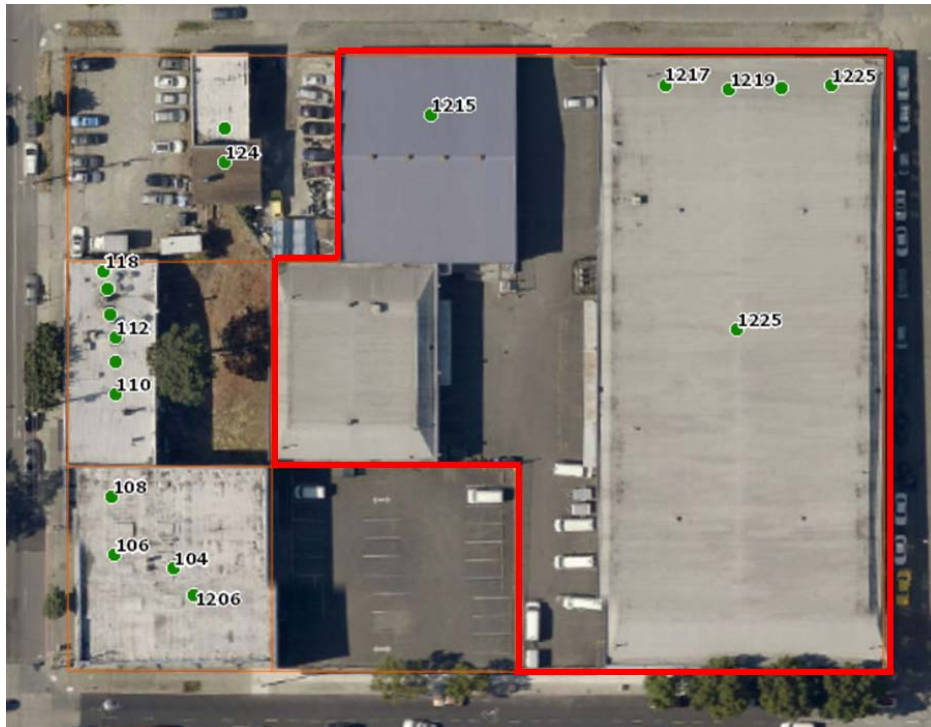
ARC – Aerial view
