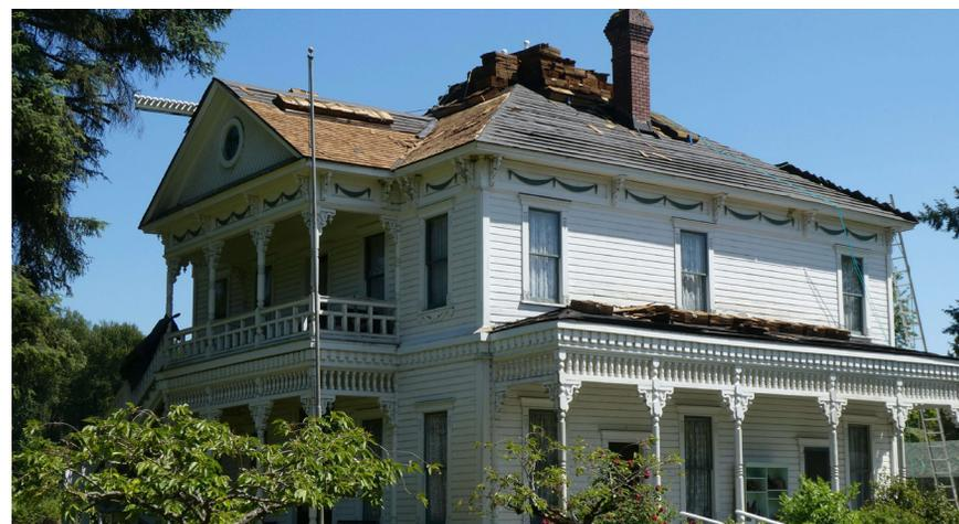
In the process of tearing off old shingles and installing new, cedar shingles, original skipjack boards were exposed on the east side of the Neely Mansion roof, 2023. Photo: Neely Mansion Association, Linda Van Nest
