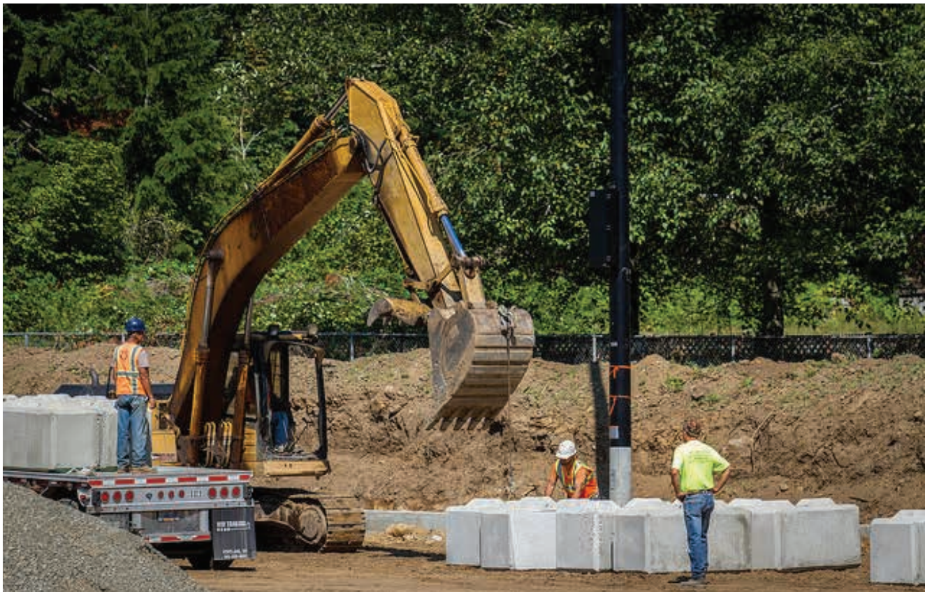
Preston Ballfields Construction
