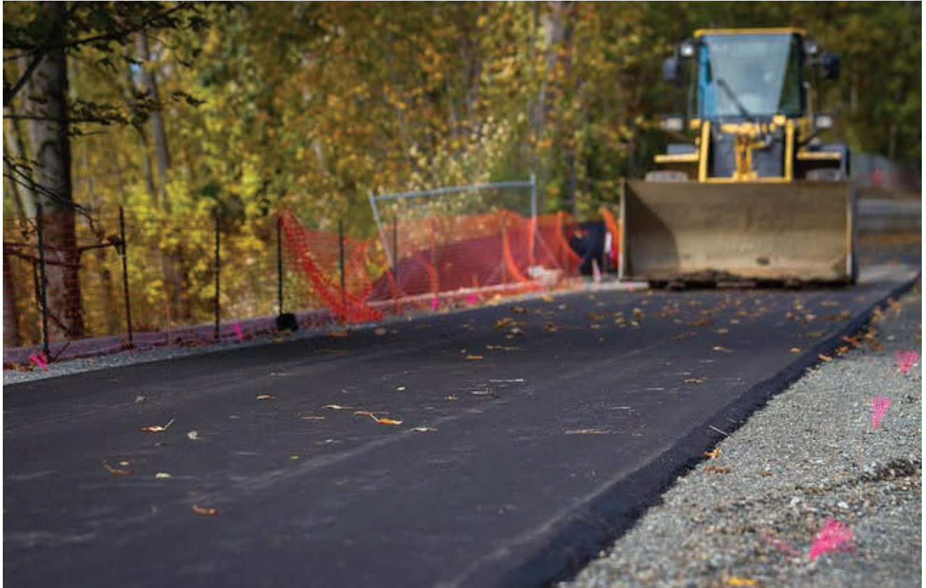
East Lake Sammamish Trail Construction
