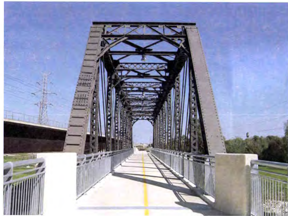
Santa Fe Trestle – Santa Fe, NM
