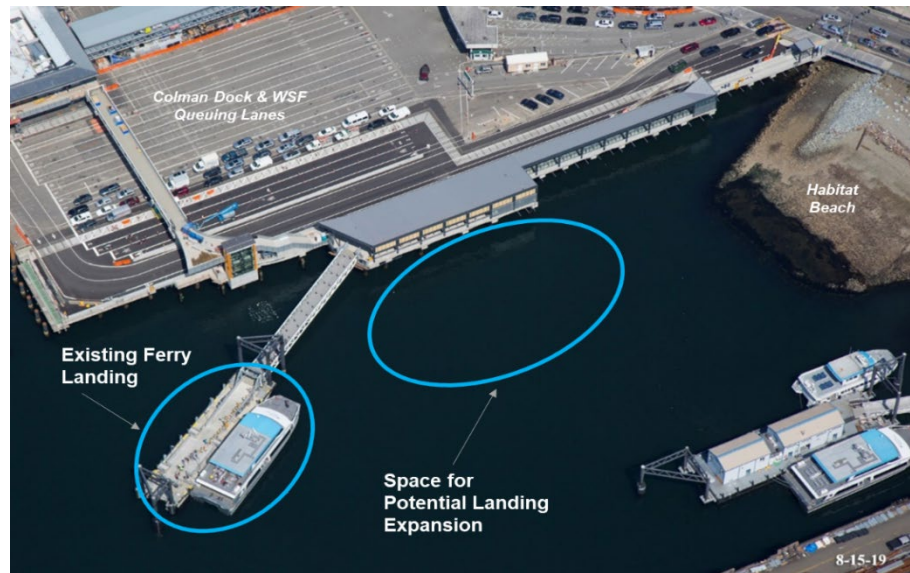
Figure 7: Aerial View of the Pier 50 Facility and Surrounding Area
