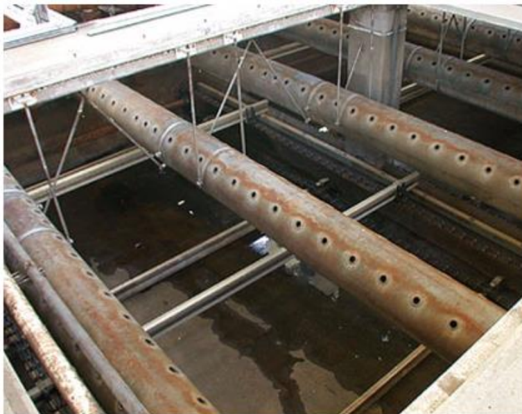
Figure 20. Effluent Launderers at the Primary Sedimentation Basins
