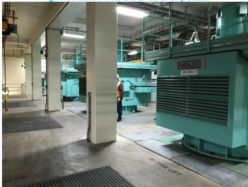
Figure 24. Electric Motors at Effluent Pump Station
