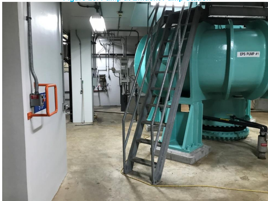
Figure 25. Pump at Effluent Pump Station
