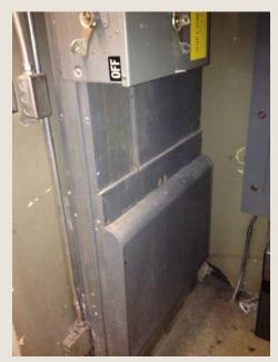
Figure 1 4000 amp buss electrical buss duct (East Riser)
