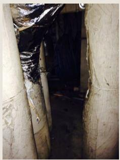
Figure 3 Access to floor 1A east electrical room (part two) by crawling through an 8" wide space between heating riser pipes. Extracting an injured worker from behind here would be next to impossible.
